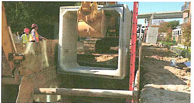
10-foot by 10-foot storm water detention boxes being installed
