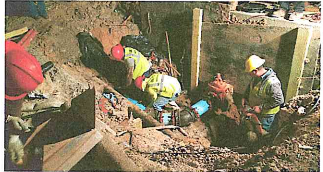
Preparing for 8-inch water line connection
