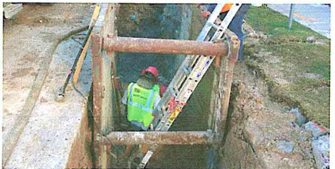
Sanitary sewer installation along Town & Country Way
