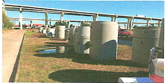
New sanitary sewer manholes stored along Town & Country Blvd.
