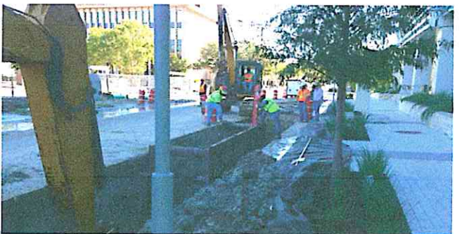
Water line installation along Town & Country Way
