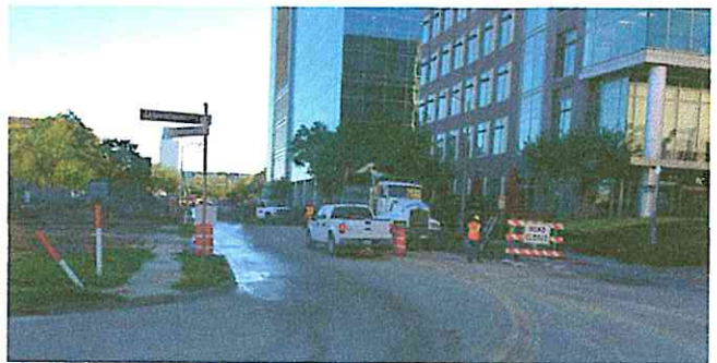
Utility work along Town & Country Way (looking east)
