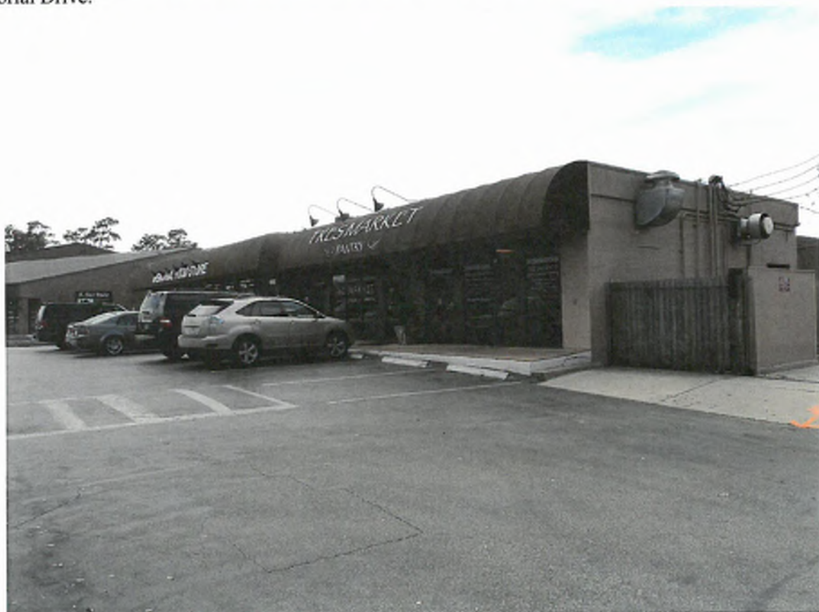
Photograph 20: View to the southwest of the former Conoco 43059 LPST site at 12699 Memorial Drive.
