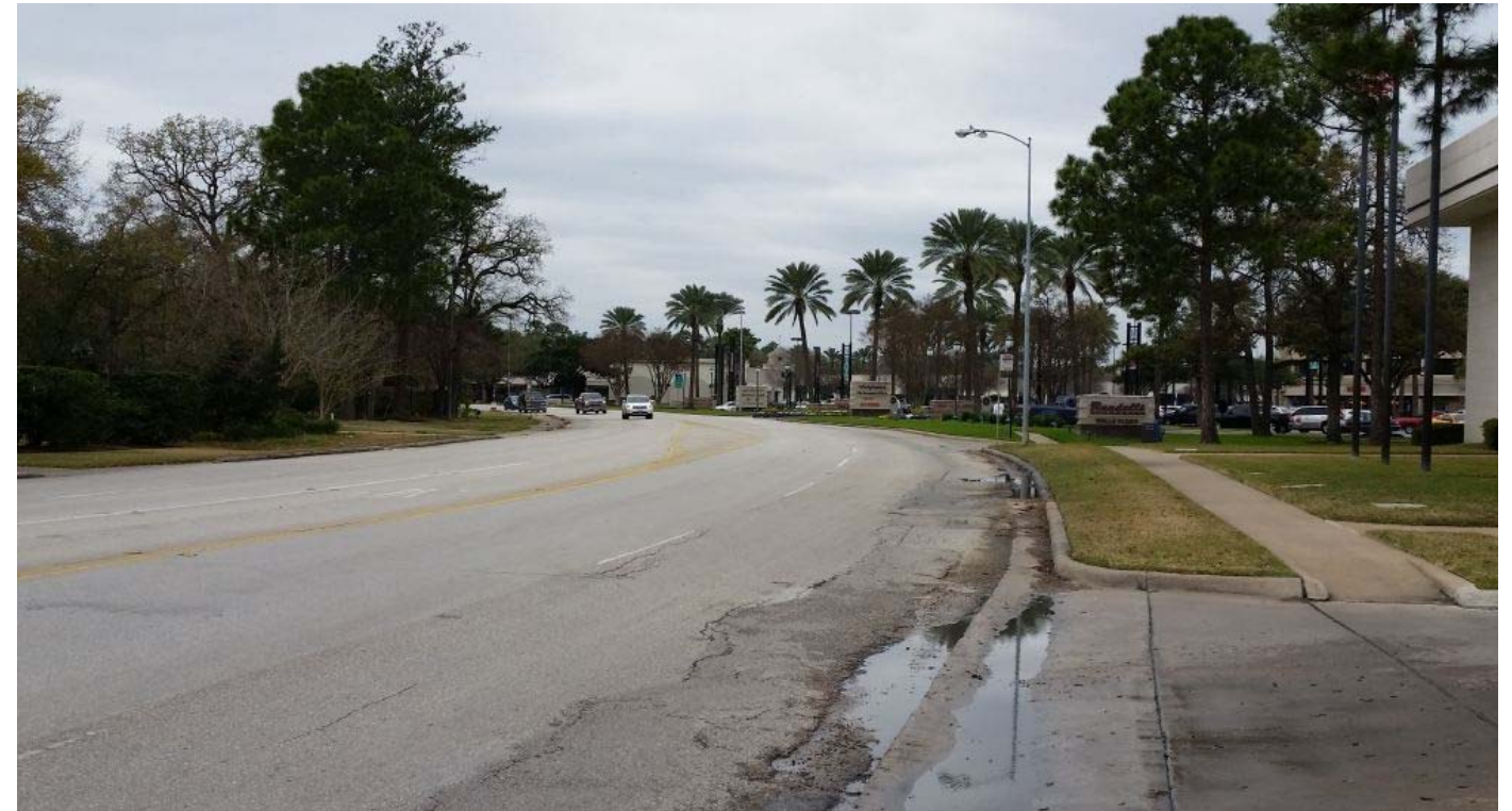
Exhibit 1.2 Memorial Drive between Beltway 8 and West Bough lane (looking west)
