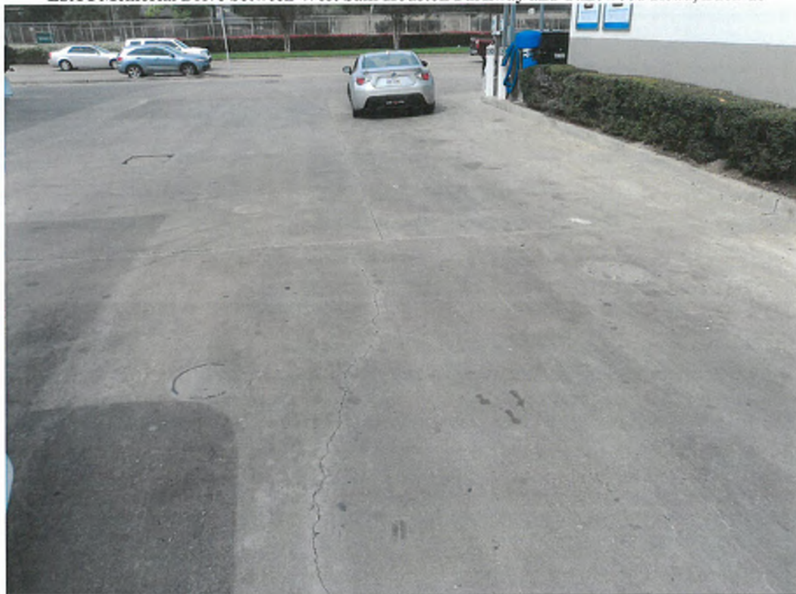
Photograph 13: View to the west of plugged monitor wells and recovery well at the Chevron LPST site.
