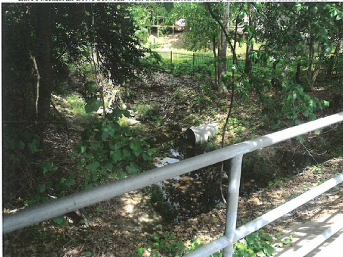
Photograph 3: View to the northwest of Harris County Flood Control District Channel W153 near Tallowood Road. The railing is the northern edge of the Memorial Drive right-of-way.
