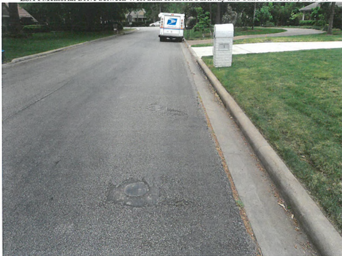
Photograph 11: View to the north towards Memorial Drive of two plugged monitor wells on Legend Lane.
