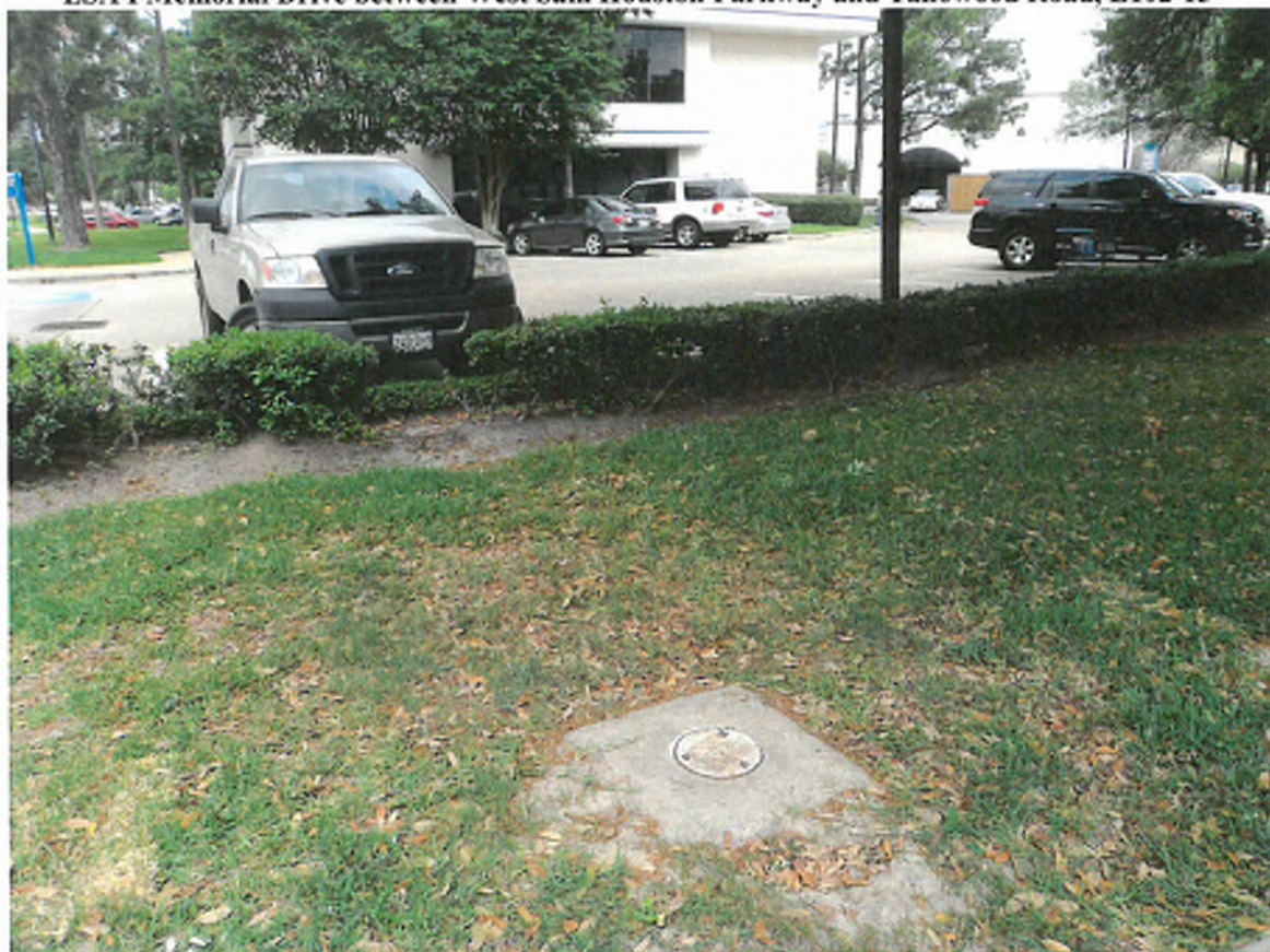
Photograph 9: View to the northwest of a monitor well on the West Bough Lane right-of-way. Chase Bank is in the background.
