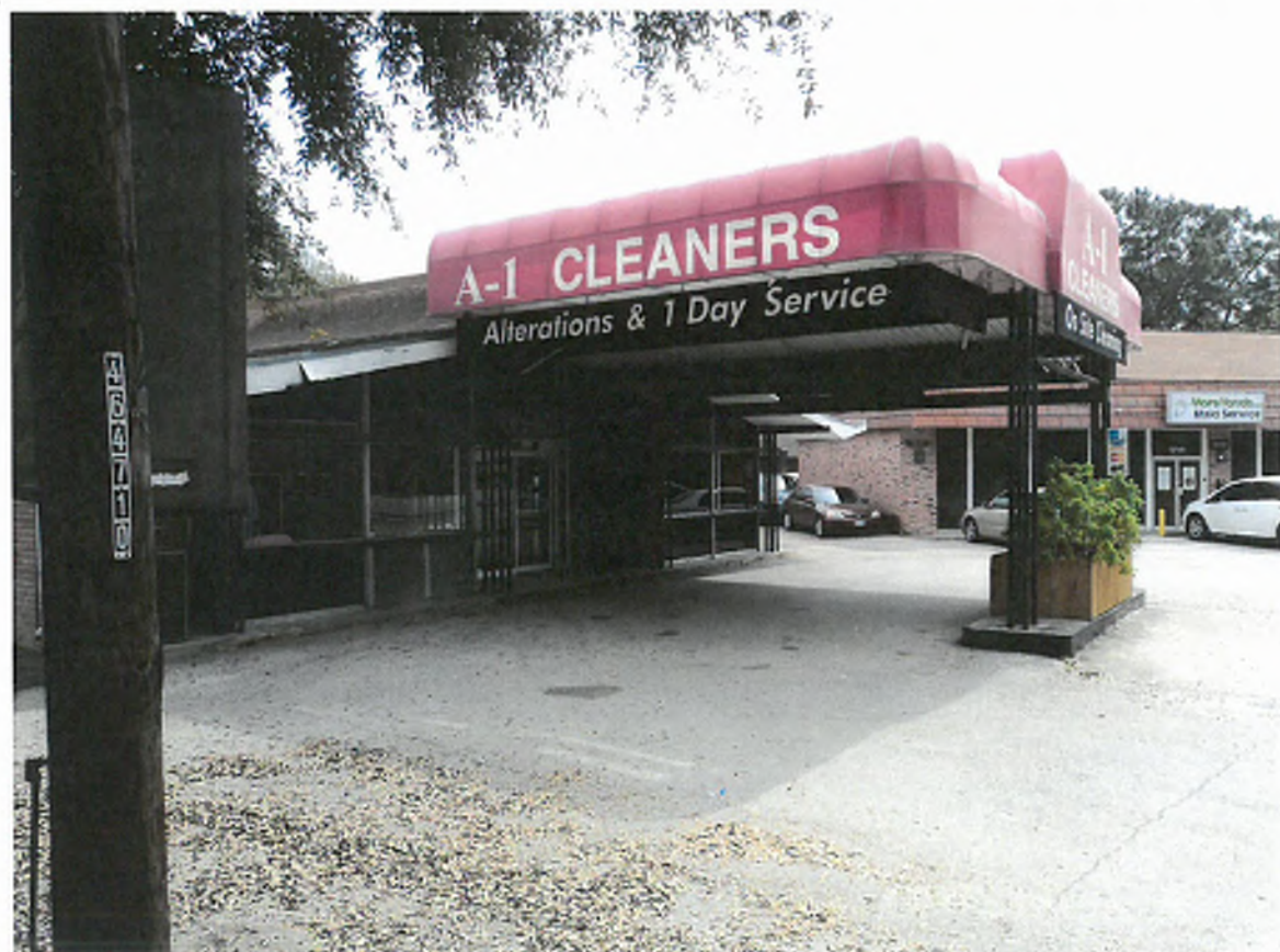
Photograph 16: View to the east of A-1 Cleaners VCP and LPST site at 12754 Memorial Drive.
