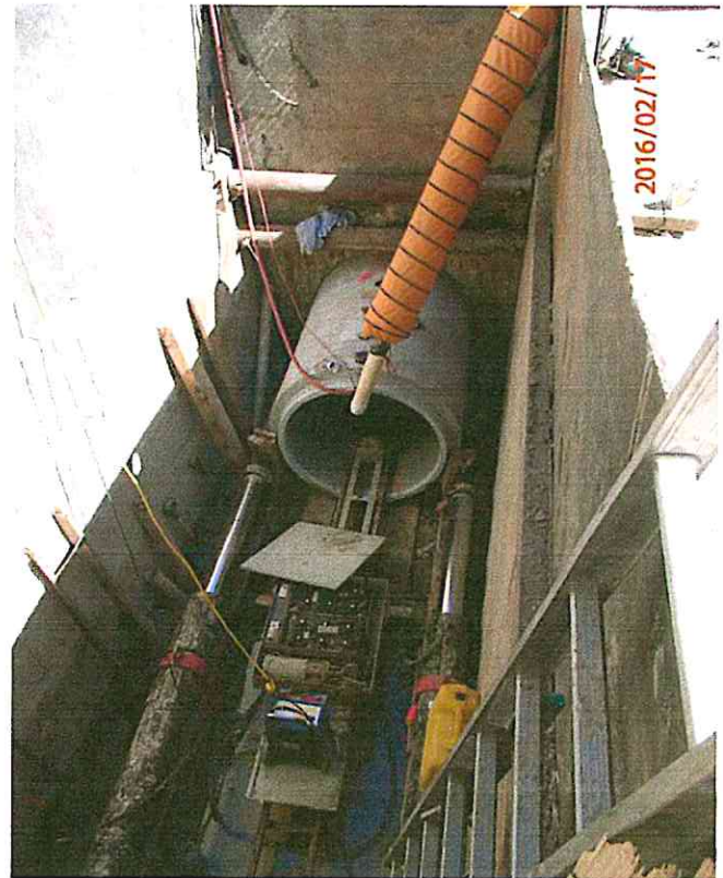
48-inch storm drain installation to Spillers Ln. cul-de-sac
