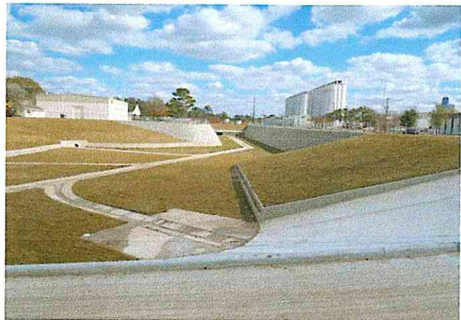
Basin looking east
