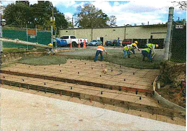
Placing new driveway
