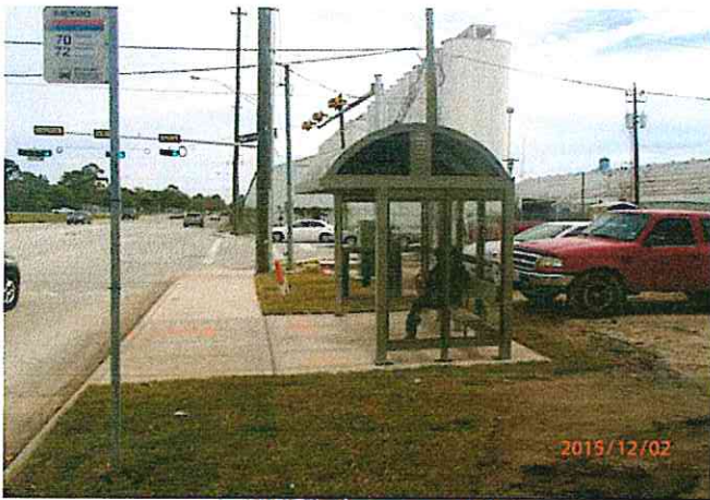
New Metro bus stop shelter
