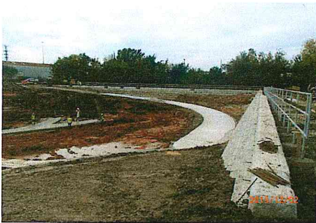
West end of basin - pilot channels, access drive and railings
