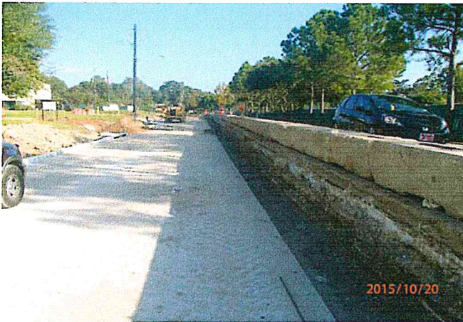
New concrete paving north of Westview Dr.
