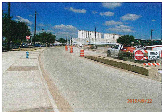
New concrete pavement along east side of Lumpkin Rd.
