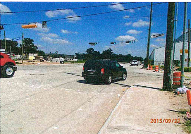
Westview Dr. east and west bound lanes opened to traffic
