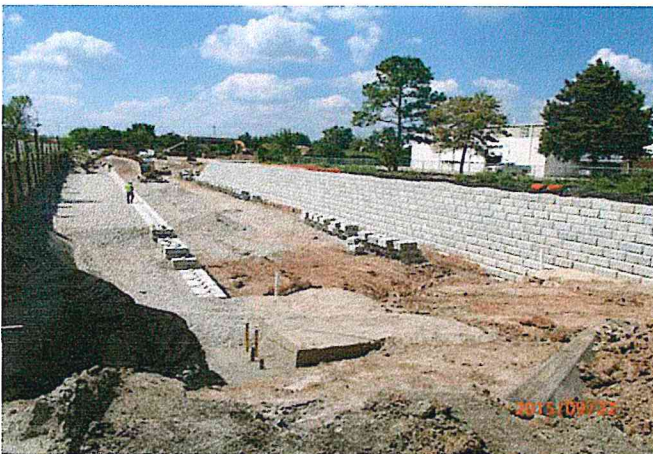
Basin modular block retaining wall installation continues
