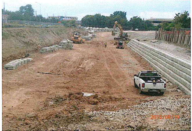
Basin modular block retaining wall installation in progress
