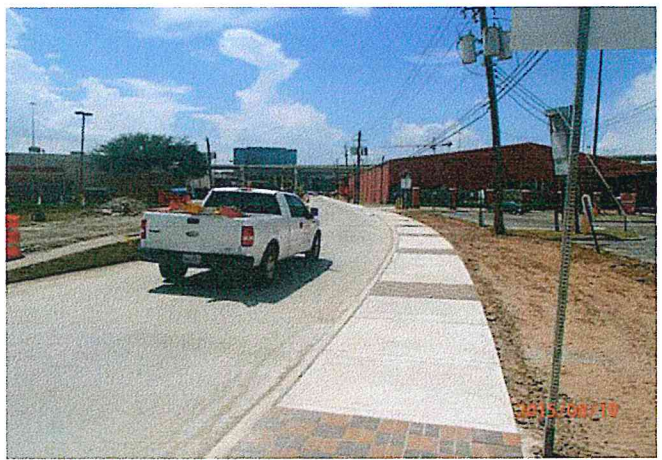
Southbound lane of Lumpkin Rd. open to traffic
