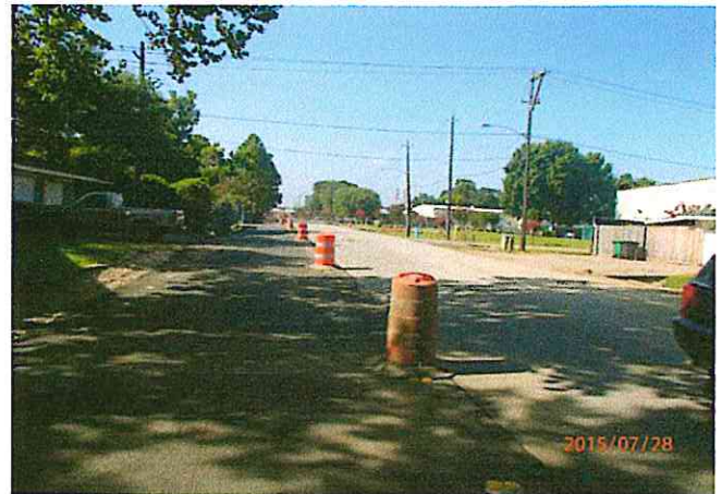
Temporary paving placed along Lumpkin Road, north of Westview Drive
