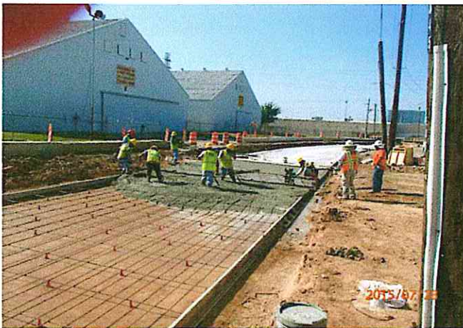
Placing concrete paving on Lumpkin Road
