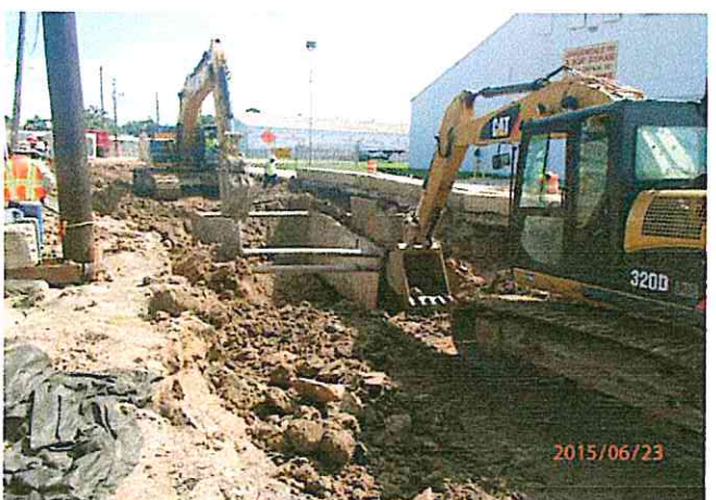
Positioning trench box for 10-ft x 6-ft storm sewer box
