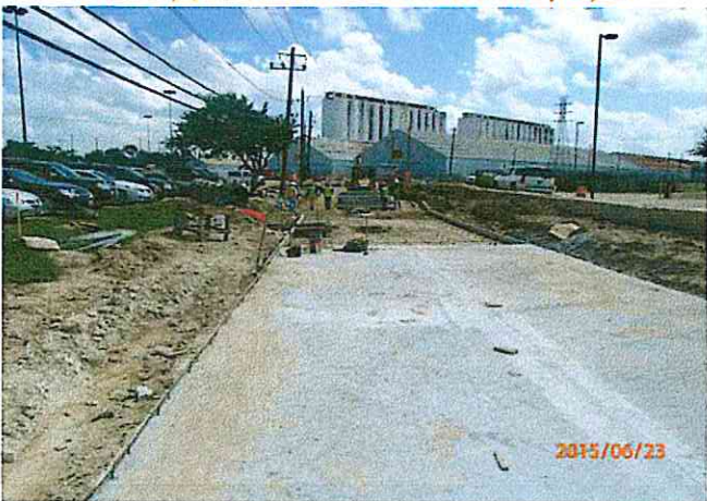
New concrete pavement installation continues
