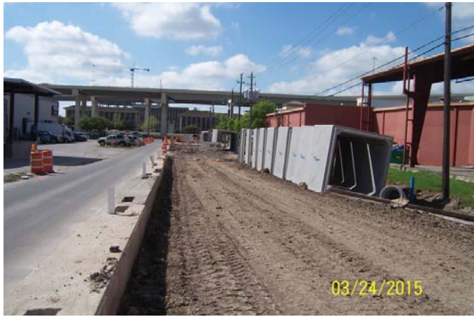
8 x 8 storm boxes staged for installation
