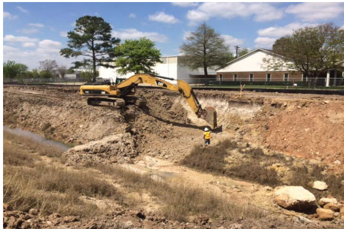
Excavating at detention basin
