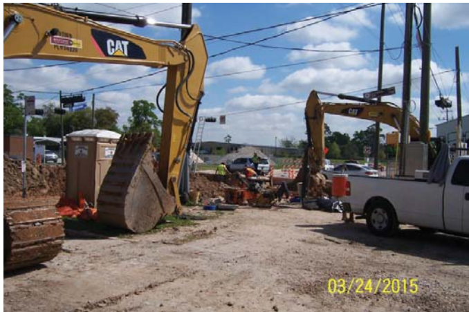
Excavation for 36-inch water line at Westview Dr.
