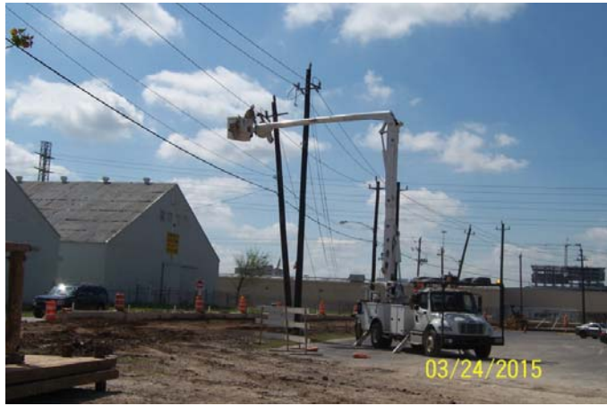
CenterPoint relocating power poles along west side of Lumpkin Rd.
