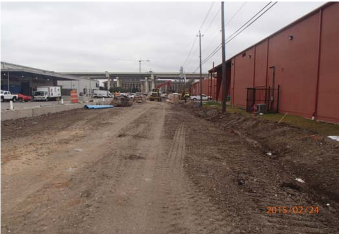
Existing paving removed for water line and storm box installation
