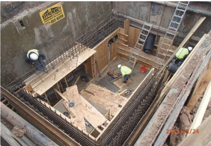
Storm junction box AM42 construction at Westview Dr.
