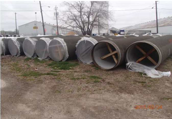
48 inch water line stored on site
