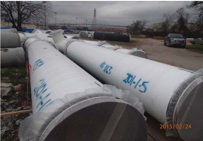
36 inch water line stored on site
