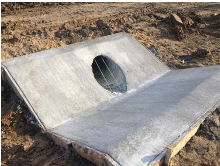
Phase II - Back slope interceptor structure with 24" outlet.
