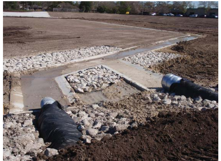
Phase II - 24" back slope drain and 36" storm sewer outfall
