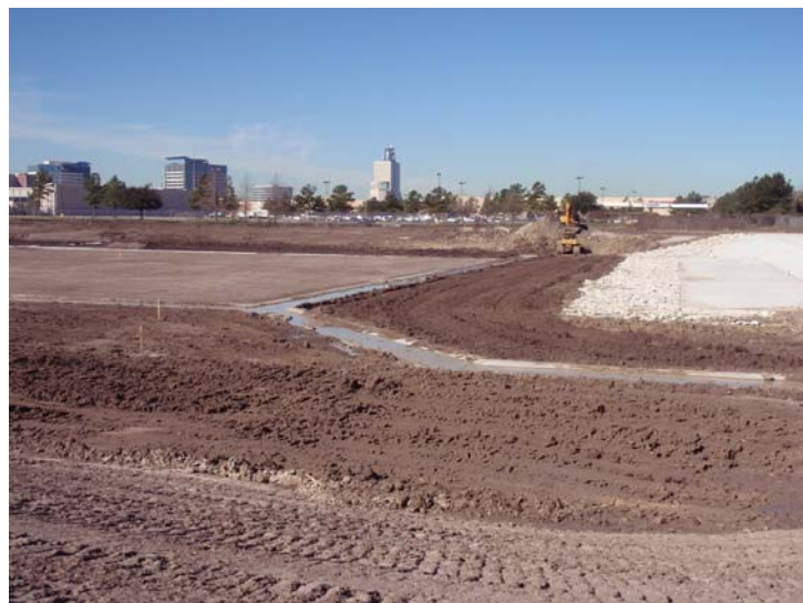
Phase II - Spreading topsoil.
