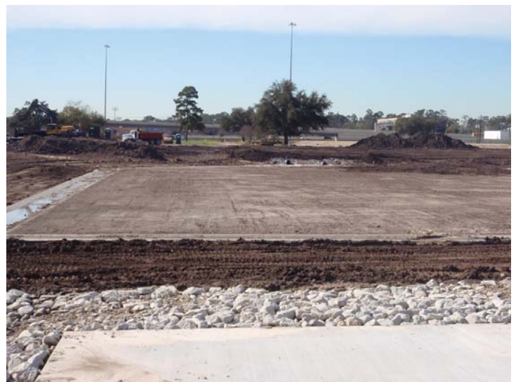
Phase II - Completing excavation at SE Corner.
