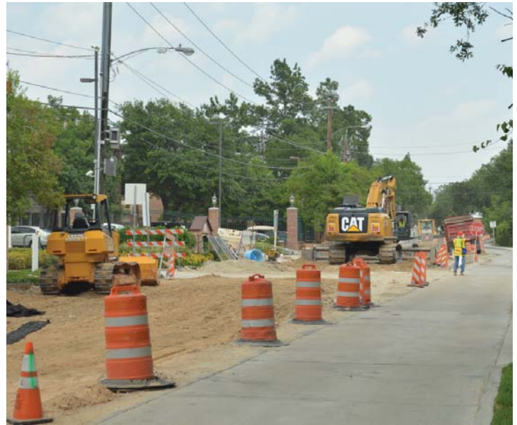
8'x6' storm sewer box installation continues east towards Bunker Hill Rd.
