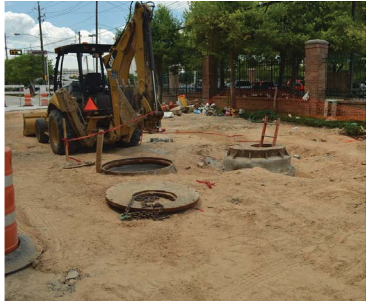
60" manholes for access to 8'x6' storm sewer boxes
