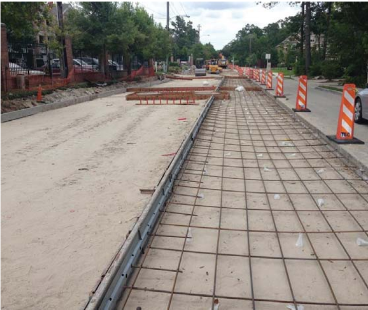
Preparing for new pavement east of Memorial City Way
