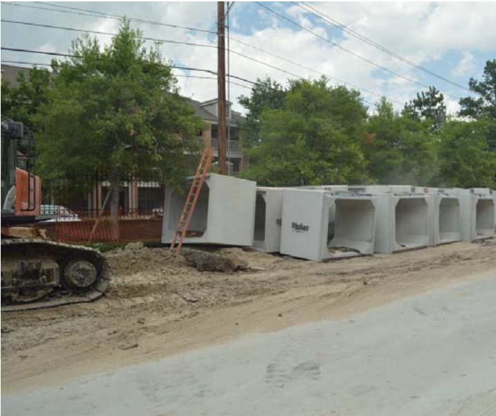
8'x6' storm sewer boxes readied for installation
