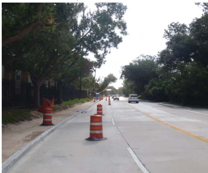
Barryknoll Lane open to two-way traffic - looking east
