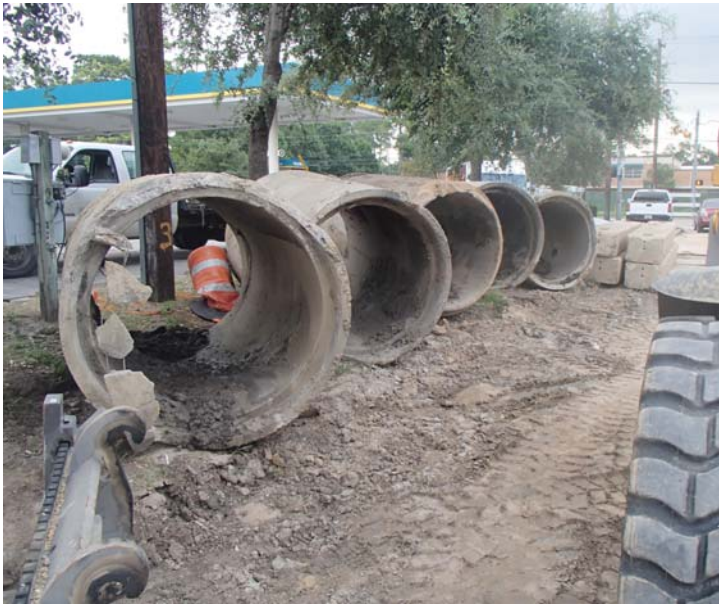
Removed section of existing 54" storm sewer pipe
