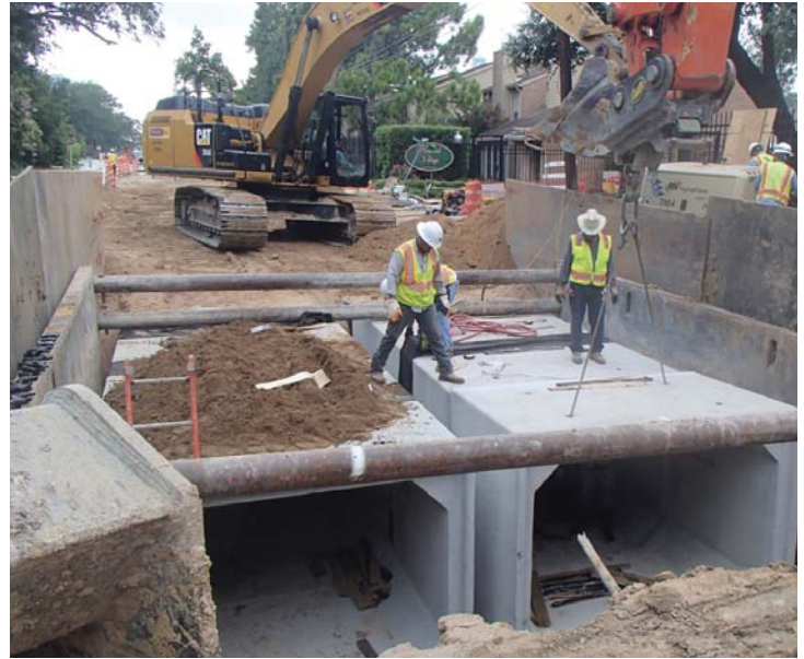
8' x 6' storm sewer box being lowered
