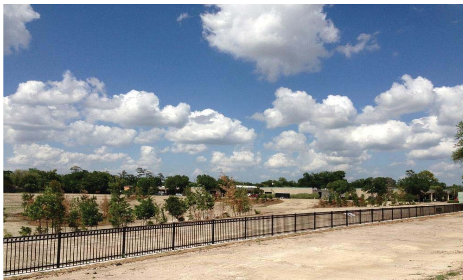
Phase II- Hydromulch, landscaping and irrigation system have been completed.
