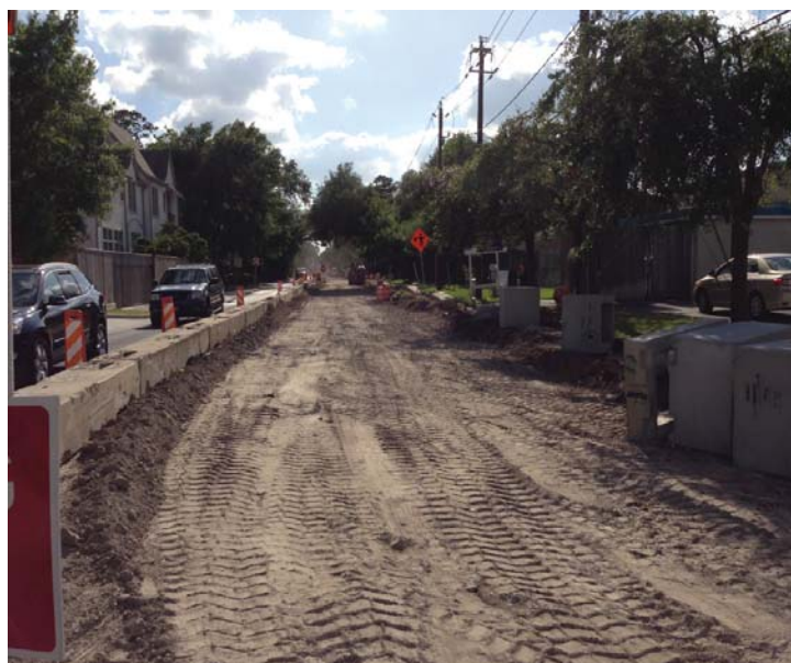
Barryknoll Lane looking west- existing paving removed.
