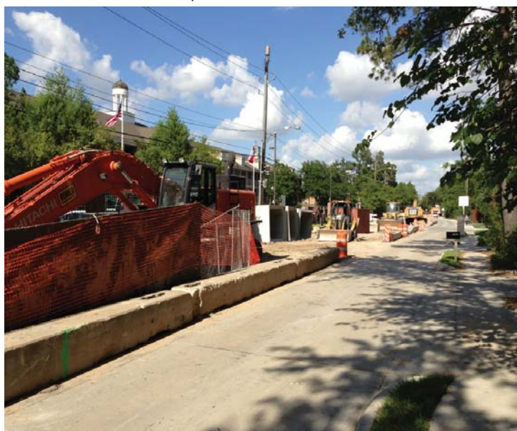
Barryknoll Lane looking east - installing storm water boxes.
