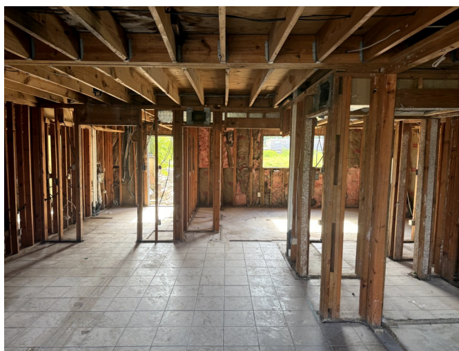
Drywall Removed—Building Ready to be Demolished
