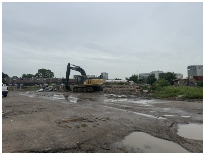
Concrete Foundation Removal
