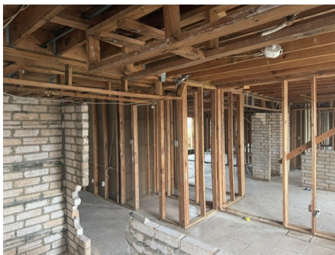
Abatement Work and Drywall Removal
