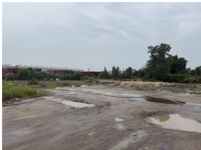
Most of Buildings are removed
