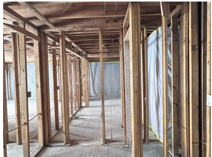
Abatement Work and Drywall Removal
