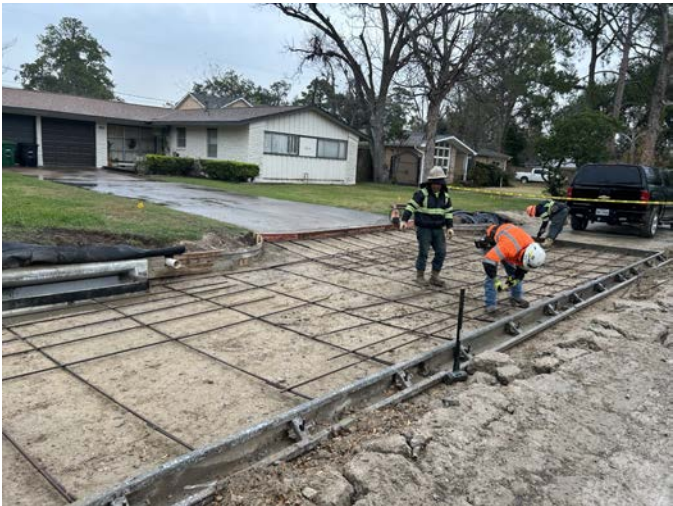
Roadway Formwork
