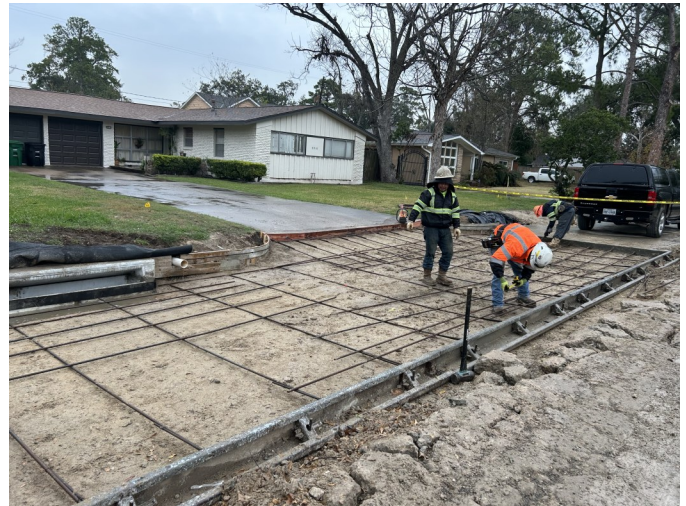
Roadway Formwork
