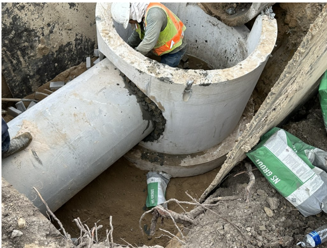
Storm Sewer Installation
