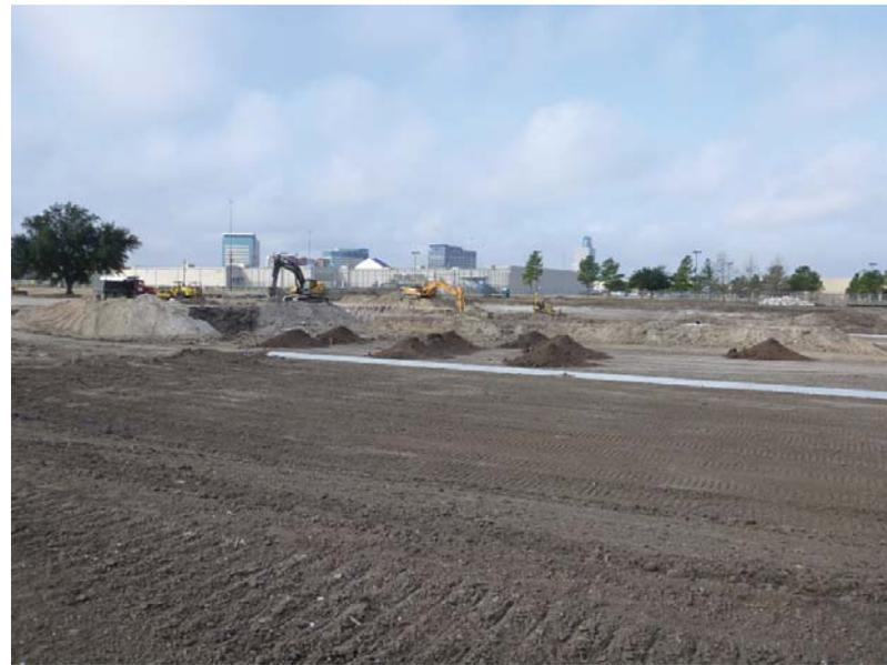
Phase II - Completing basin excavation at south end.
