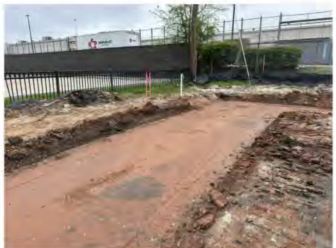
Slurry Wall Cap Installation
