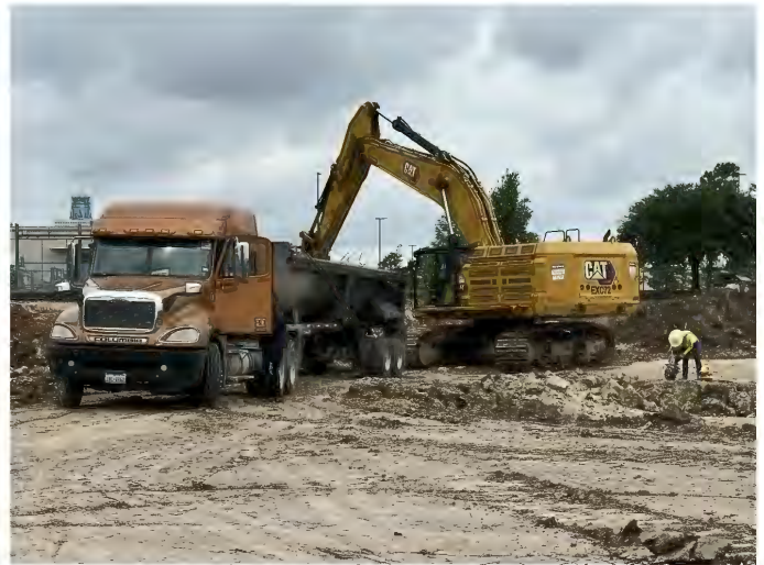
Excavation and Offsite Disposal
