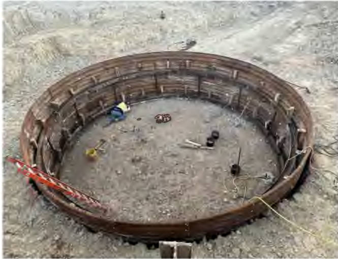
Liner Plate Shaft Installation for Wet Well
