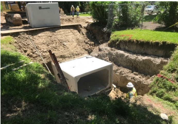
Box Installation—Long Branch & W140-01-05 (Straw 5)
