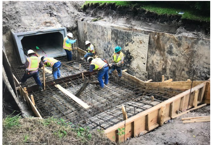
Forming flooring - Long Branch & W140-01-05 (Straw 5)
