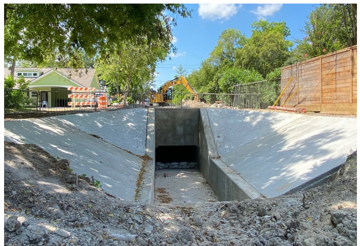
Final wing and head wall structure ( Straw 5)
