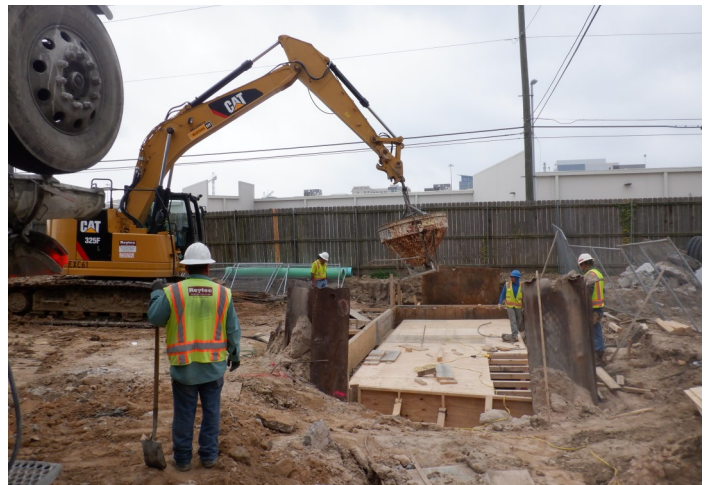
Pouring concrete at Junction Box.
