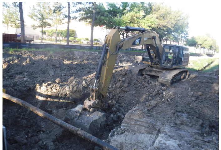
Removal of concrete channel lining
