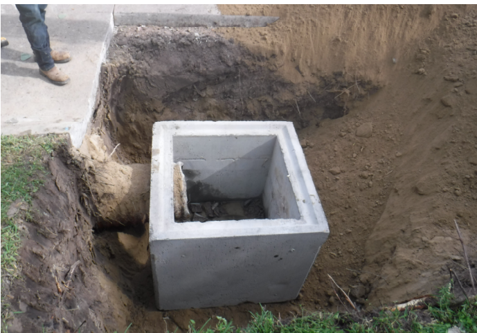
Installation of C-1 inlet along Larston @ Cederdale
