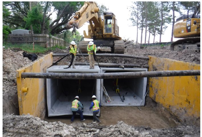
10' x 8' and 9' x 8' RCB Installation—PH I
