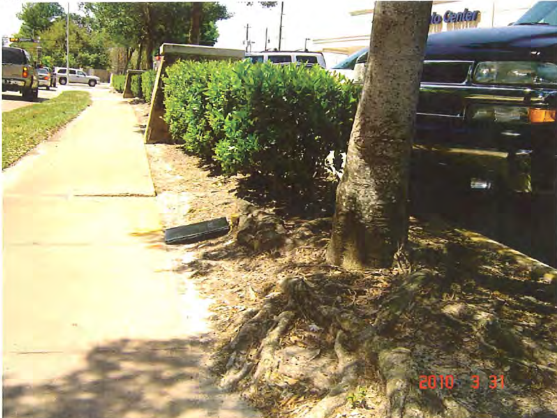
Figure 3: Iron rod at right of way and root mass at north side of walk at tree 11.
