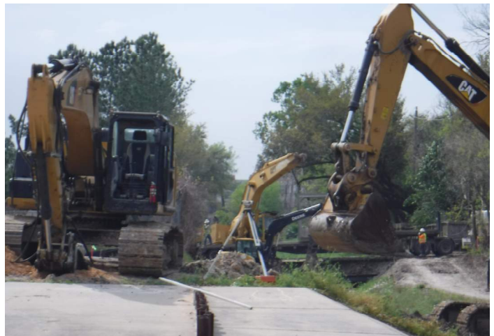
Prep work for 9' x 8' RCB Installation—PH I
