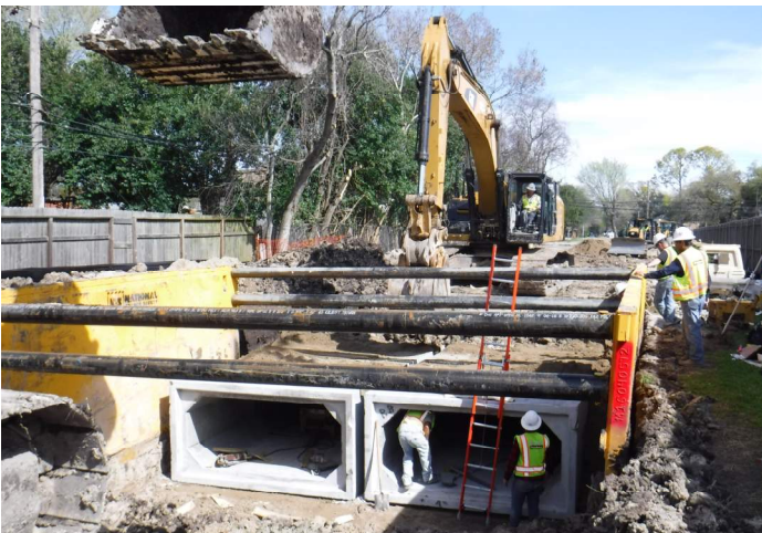
8' x 4' RCB Installation — PH III
